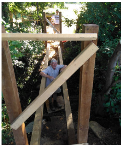
End of day 1 - beams and uprights in place and temporary bracing
